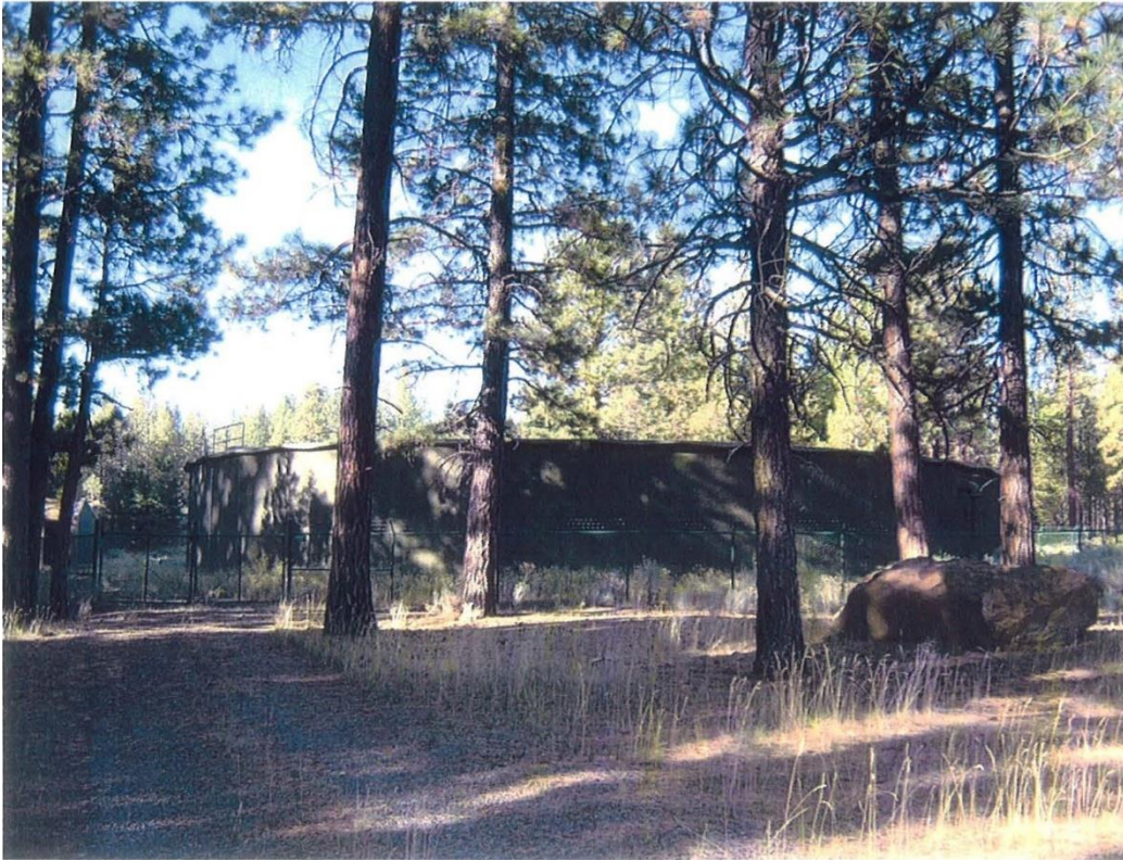
Figure 3. 3: Existing 1.6 Million Gallon Reservoir
