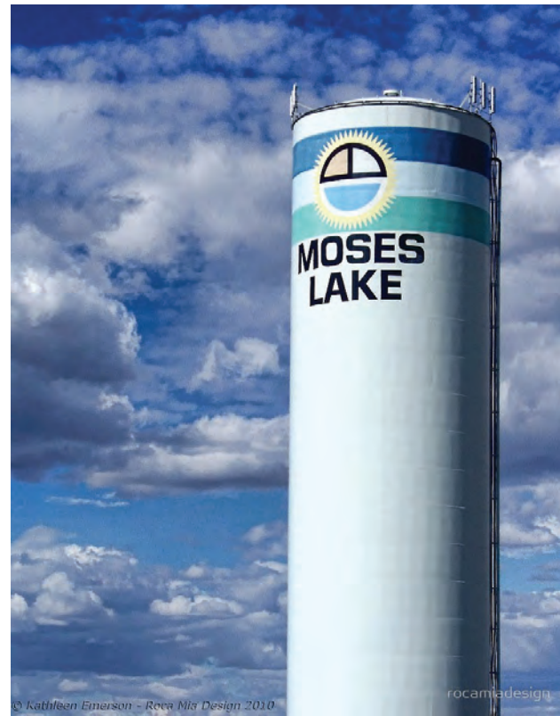
Standpipe Style Welded Steel Reservoir Moses Lake, Washington (courtesy of Rocamia Design)
