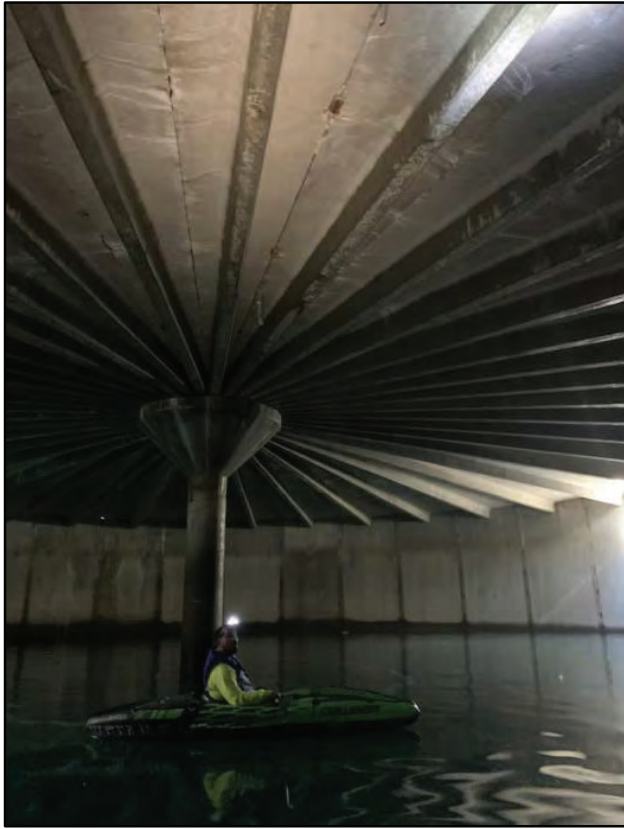
Figure 7: Interior view – Float inspection
