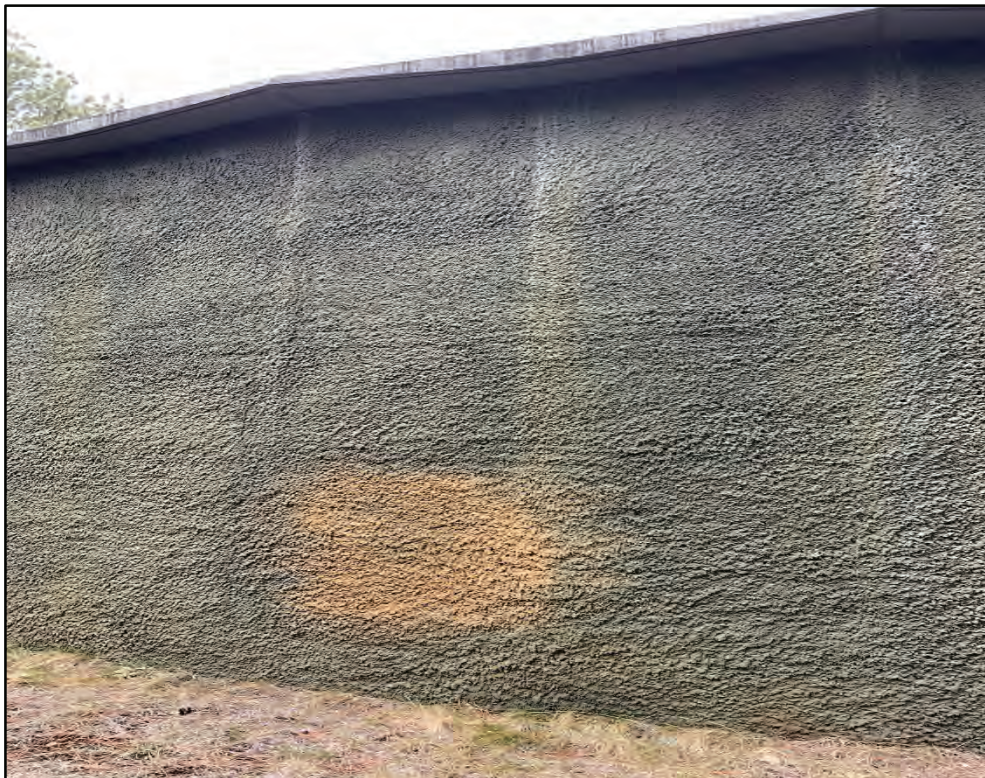
Figure 2: Exterior View of Reservoir Wall
