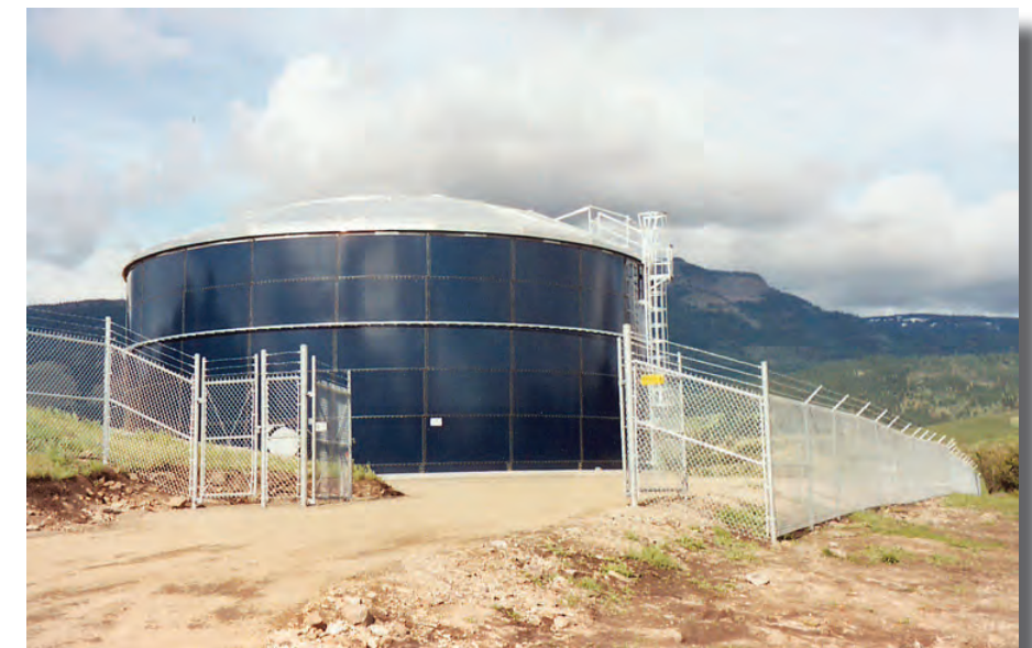
Ground Level Bolted Steel Reservoir - Cove, Oregon
