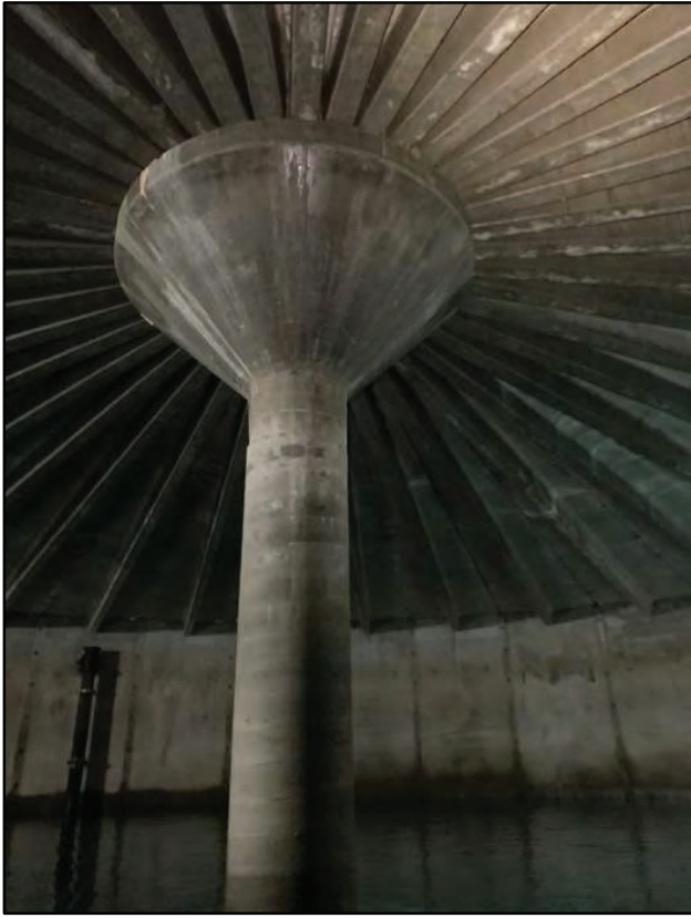
Figure 9: Interior View of Column
