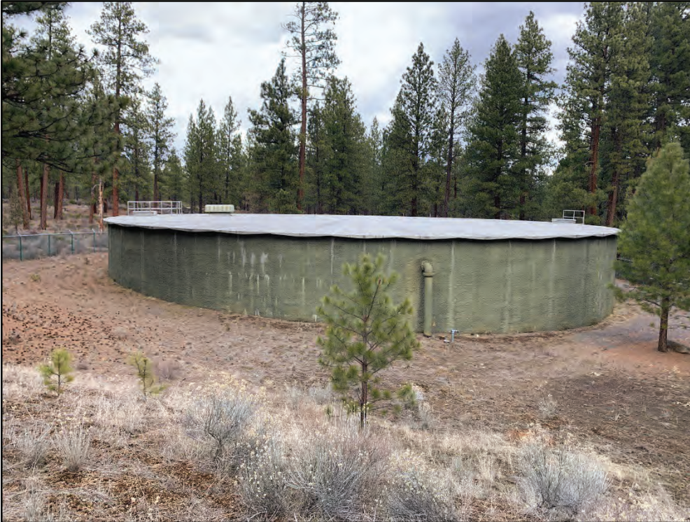
Figure 1: Exterior View of Reservoir
