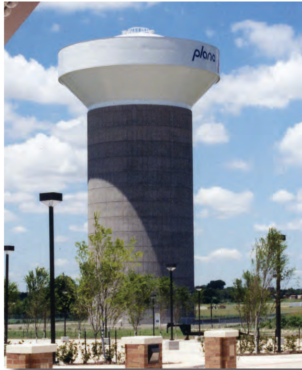
Pillar Style Elevated Composite (Concrete/Steel) Reservoir - Plano, Texas (Courtesy of CB&I)
