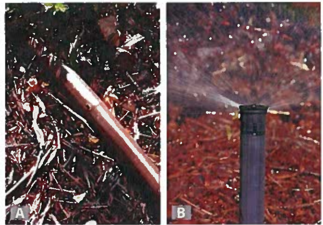
Figure 4. For trees, shrubs, and perennials, use a dripline (A), pop-up irrigation (B), or microsprays.
