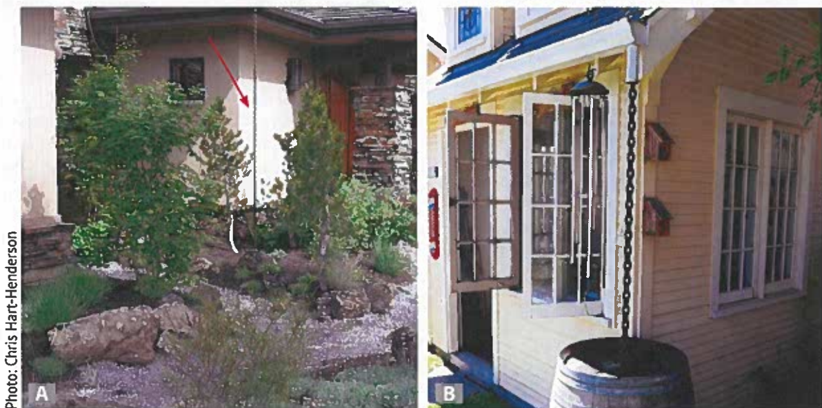
Figure 3. Rain chains are practical tools to help manage stormwater runoff by diverting water to where it will benefit the garden (A) or collecting it in cisterns or barrels so that it can be used later for irrigation (B).
