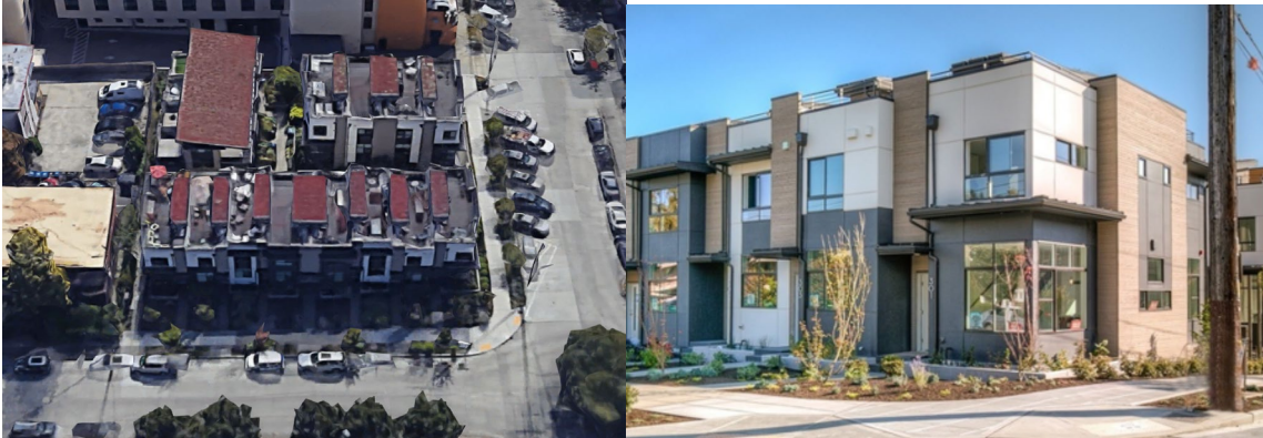
Above: Townhouses and Live/Work Units in Seattle WA at 44 DU/Net Acre
