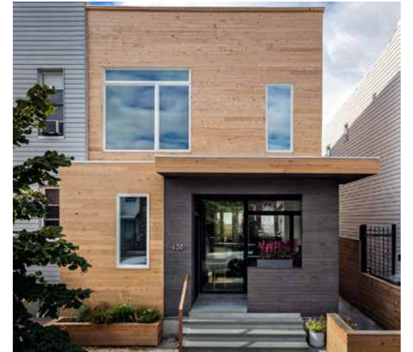
BFDO Architects - 20th Street House
