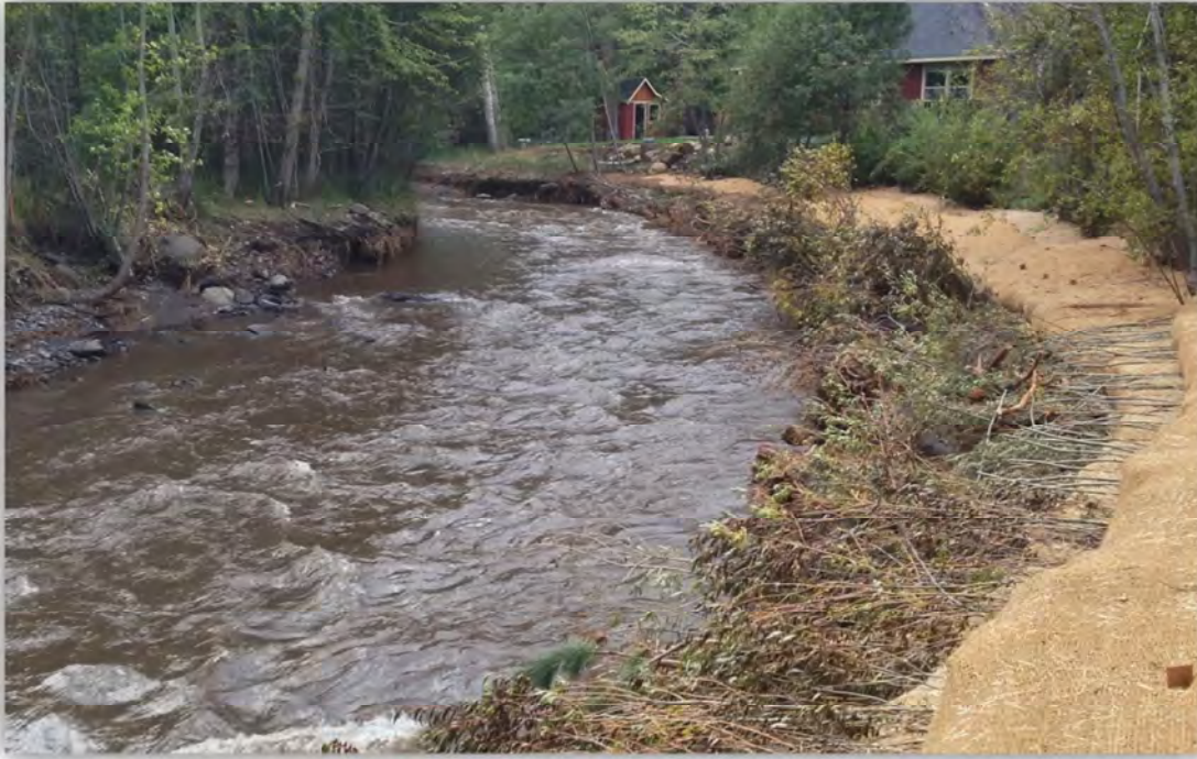
Figure 5: Example of a Bio-Engineered Soil Lift (Photo Taken Immediately Upon Completion)
