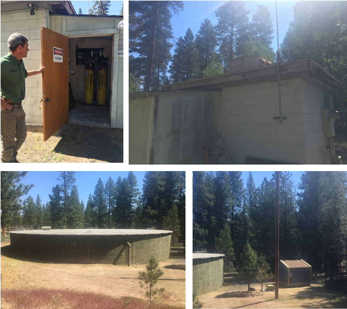
Figure 13. Well #1 (top) has unique vulnerabilities to wildfire that require mitigation strategies. Specific vulnerabilities include the storage of chlorine gas. Fire damage to the well structure that affects the gas tanks may lead to well contamination, chlorine exposure, or malfunction of water treatment systems. Concerns related to the city's reservoir (bottom) include restricted access during a wildfire event to ensure an ongoing power supply is maintained. Images source: CPAW
