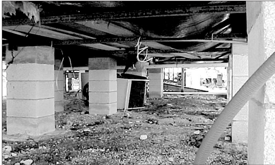
Figure 1-4. Reinforced masonry pier foundation system under a manufactured home installed after 1994 that performed well.
