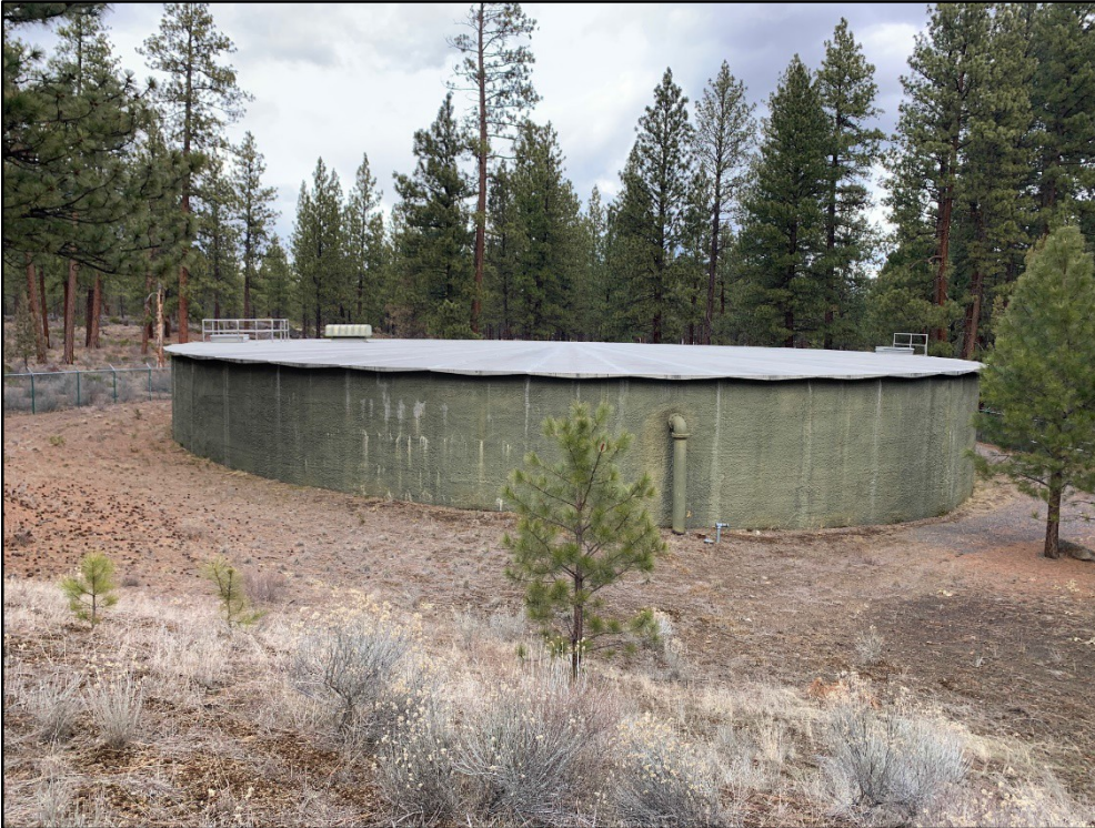
Figure 1: Exterior View of Reservoir
