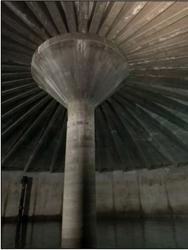
Figure 9: Interior View of Column
