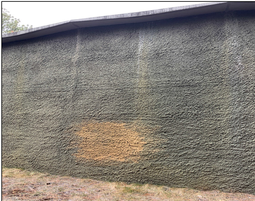
Figure 2: Exterior View of Reservoir Wall
