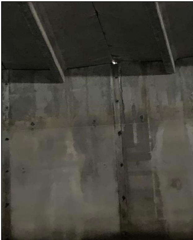
Figure 10: Interior view – Note potential daylight – found in several locations
