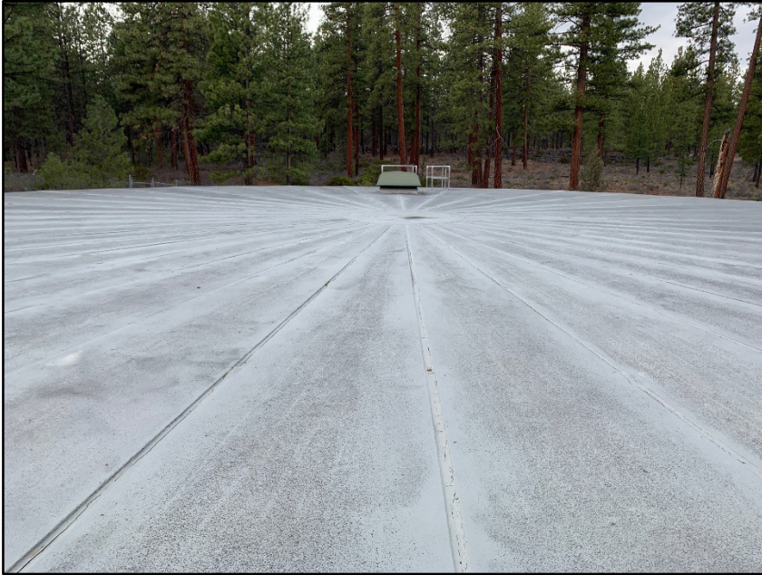
Figure 11: Exterior Roof – Note construction joints and existing coating
