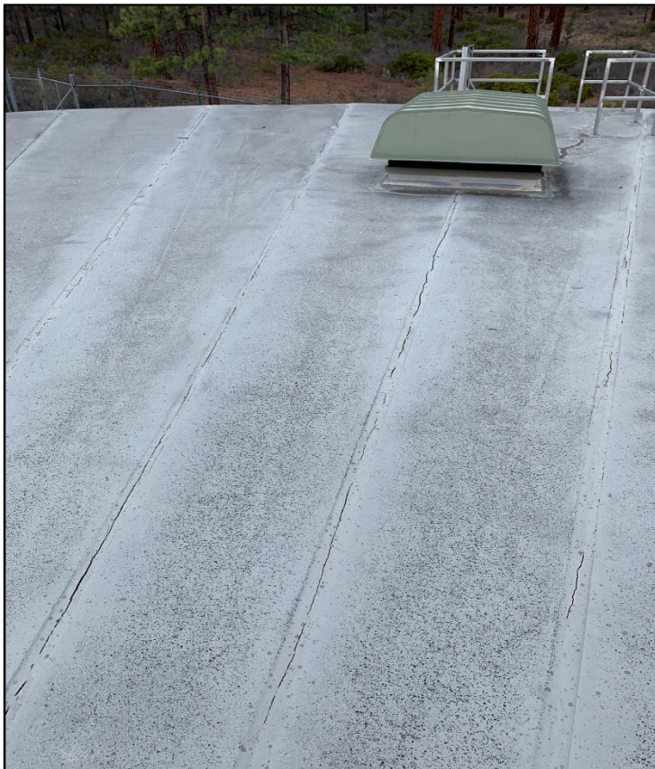
Figure 11: Exterior Roof – Note construction joints and existing coating
