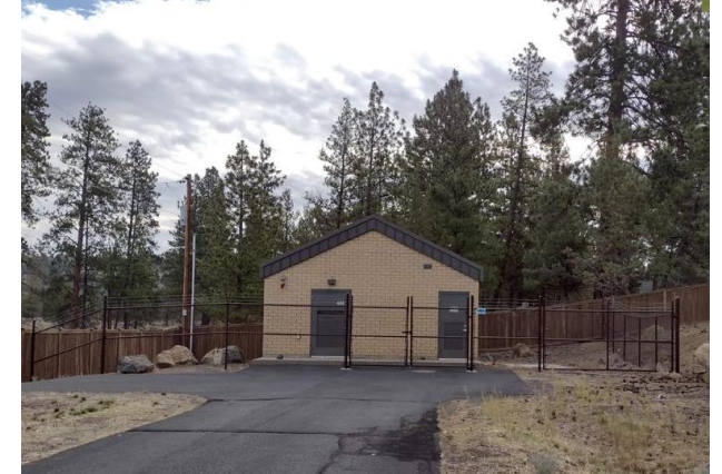
Rope Street Lift Station
