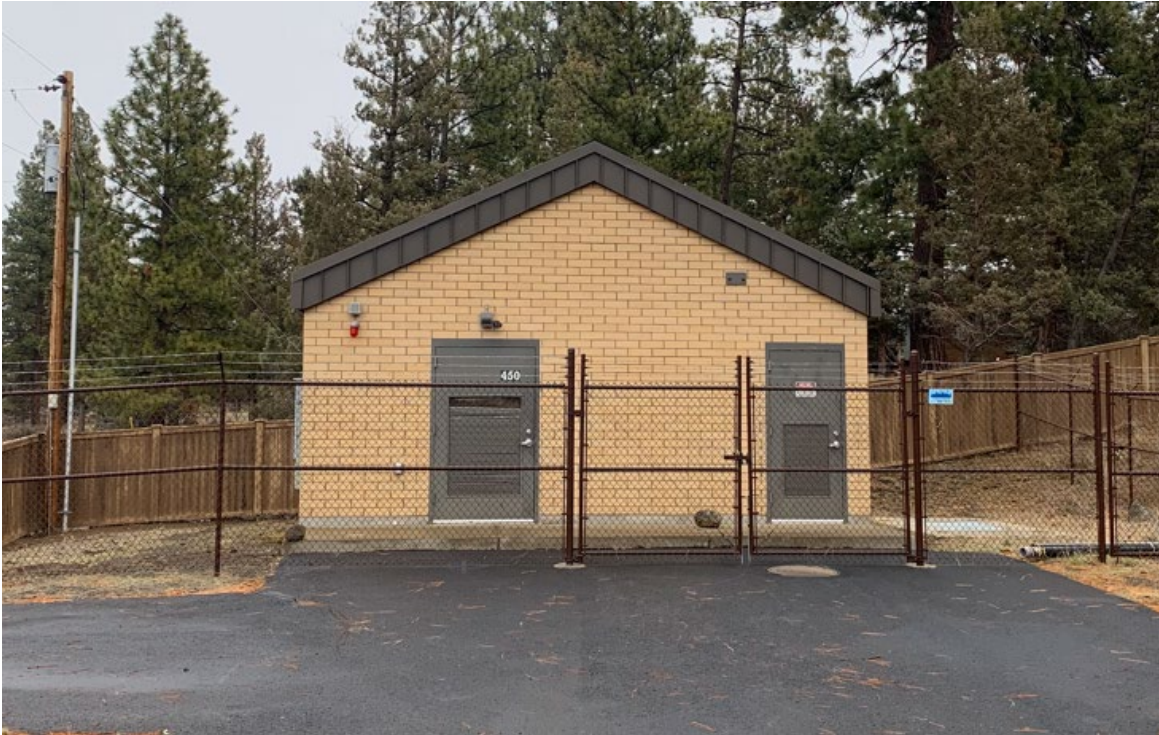
Rope Street Pumpstation
