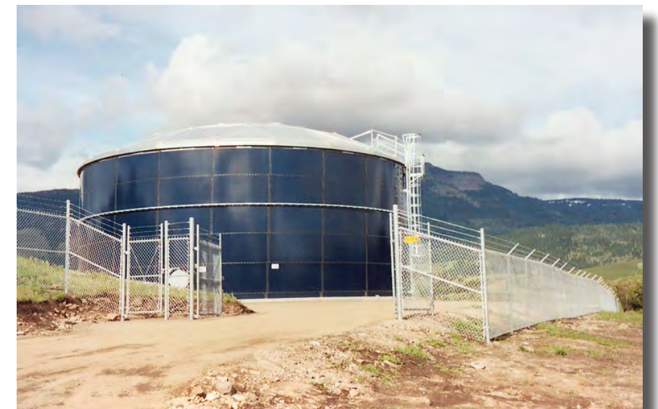
Ground Level Bolted Steel Reservoir - Cove, Oregon
