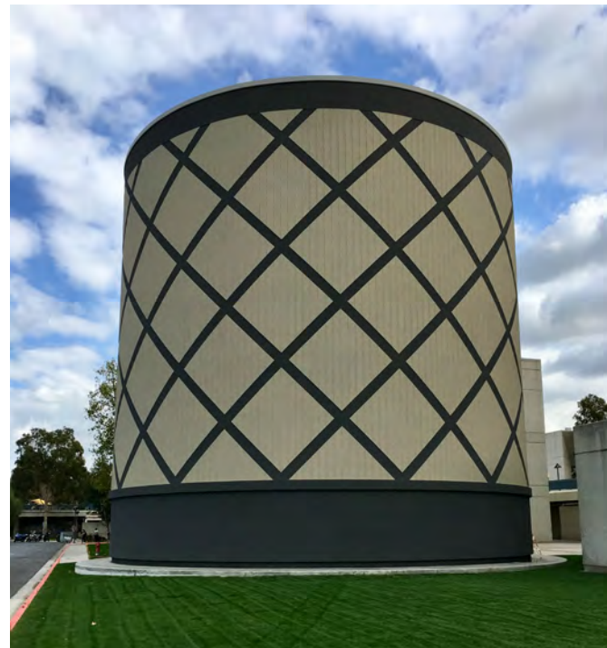
Prestressed Concrete Reservoir Cypress College in Cypress, CA (courtesy of DN Tanks)
