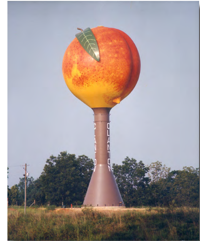
Spherical Elevated Steel Reservoir Clanton, Alabama (Courtesy of CB&I)
